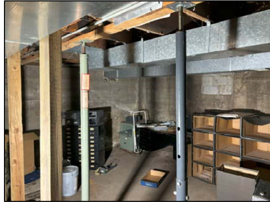
Photo 60: General view of the support beams holding the floor up
