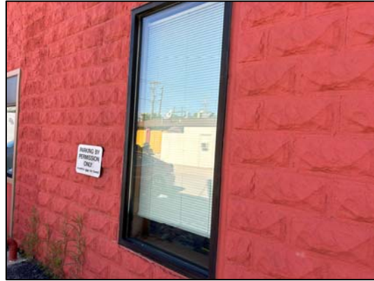
Photo 4: General view of the new commercial windows
