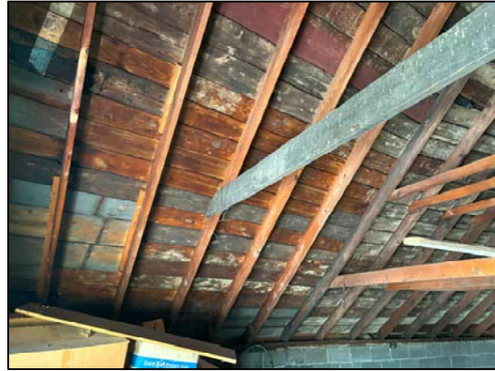
Photo 20: General view of the old wooden boards beneath the shingles
