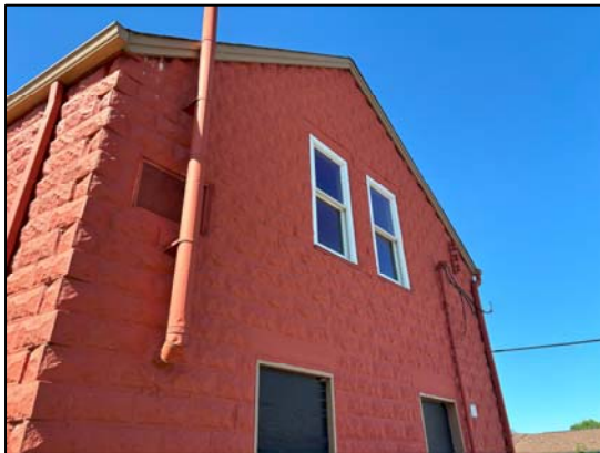
Photo 8: General view of the ventilation pipe
