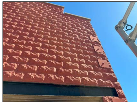
Photo 12: General view of the wall supports along the south wall
