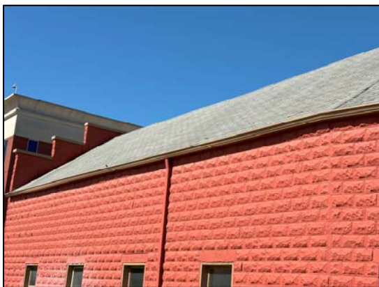
Photo 19: General view of the gutter system along the east wall
