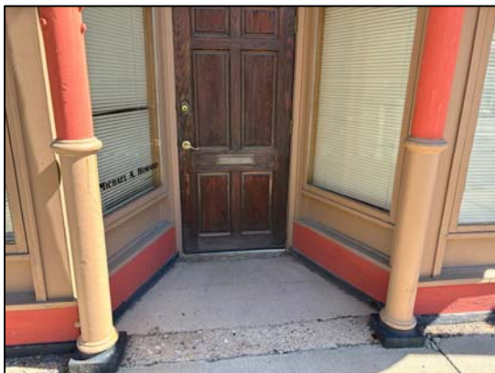
Photo 15: General view of the south main entrance
