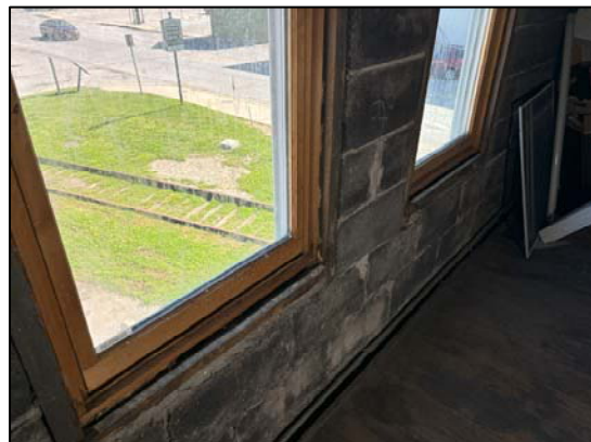
Photo 50: General view of the older wooden framed windows upstairs
