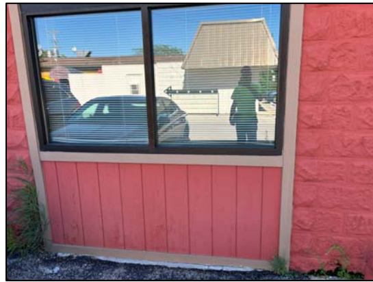
Photo 5: Another view of the new commercial windows
