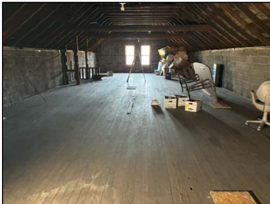
Photo 52: General view of the upstairs flooring
