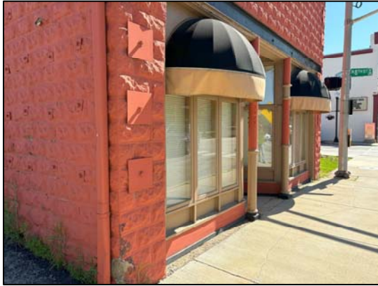
Photo 1: General view of the Subject Building
