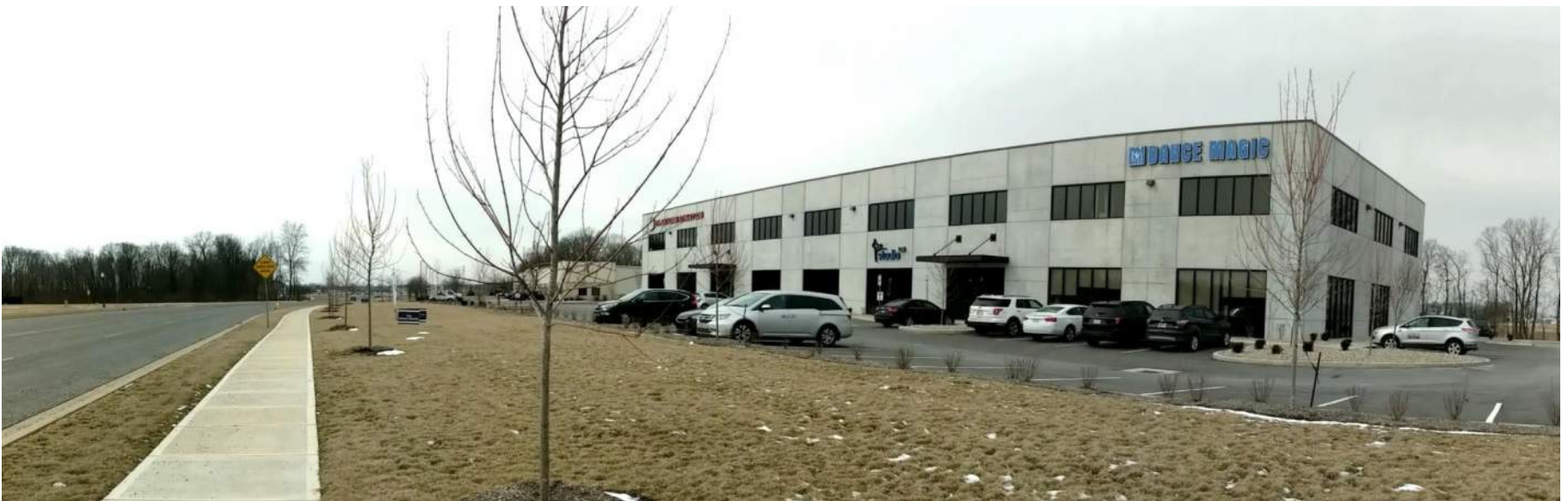
Looking northwest to the south building elevation along Pleasant Street.
