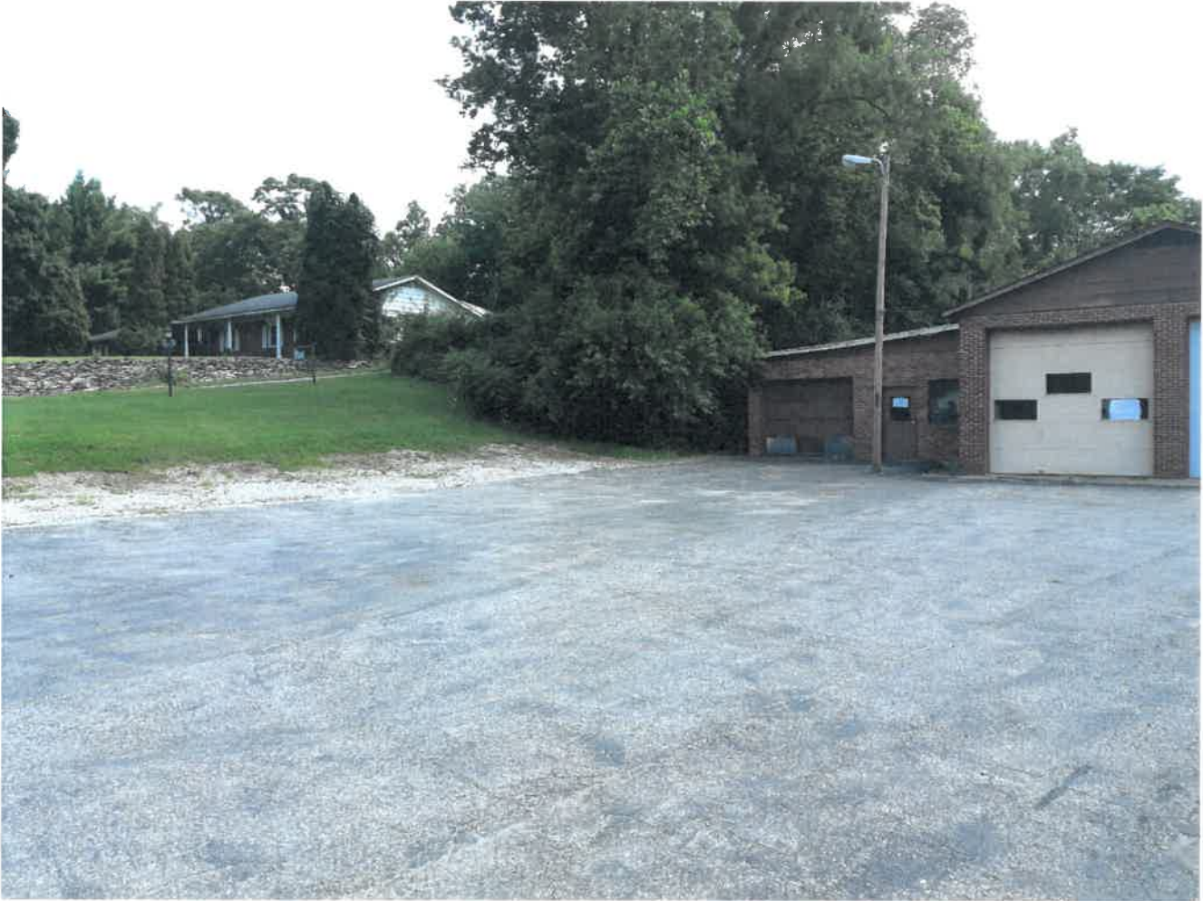
Looking northeast toward single-family residence on same parcel
