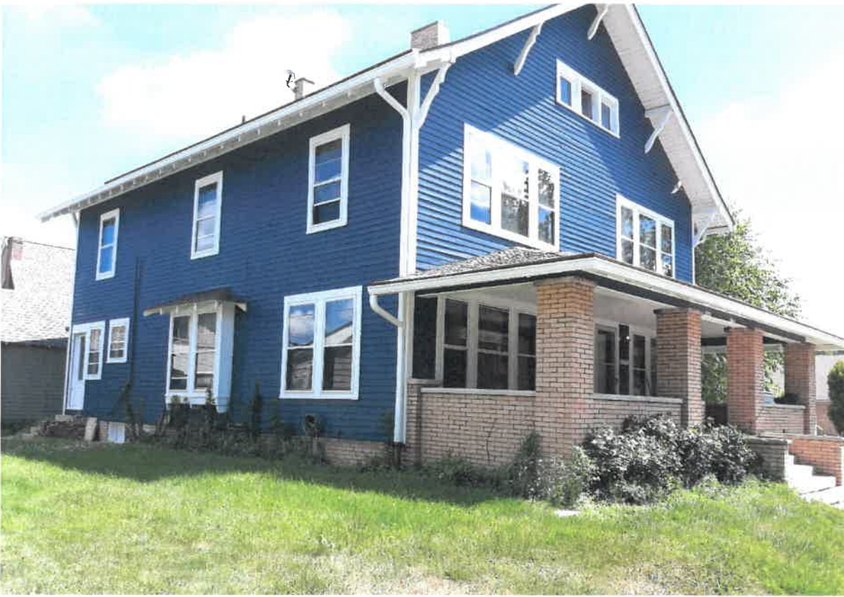
Photo 1: View from Logan Street, looking northeast
