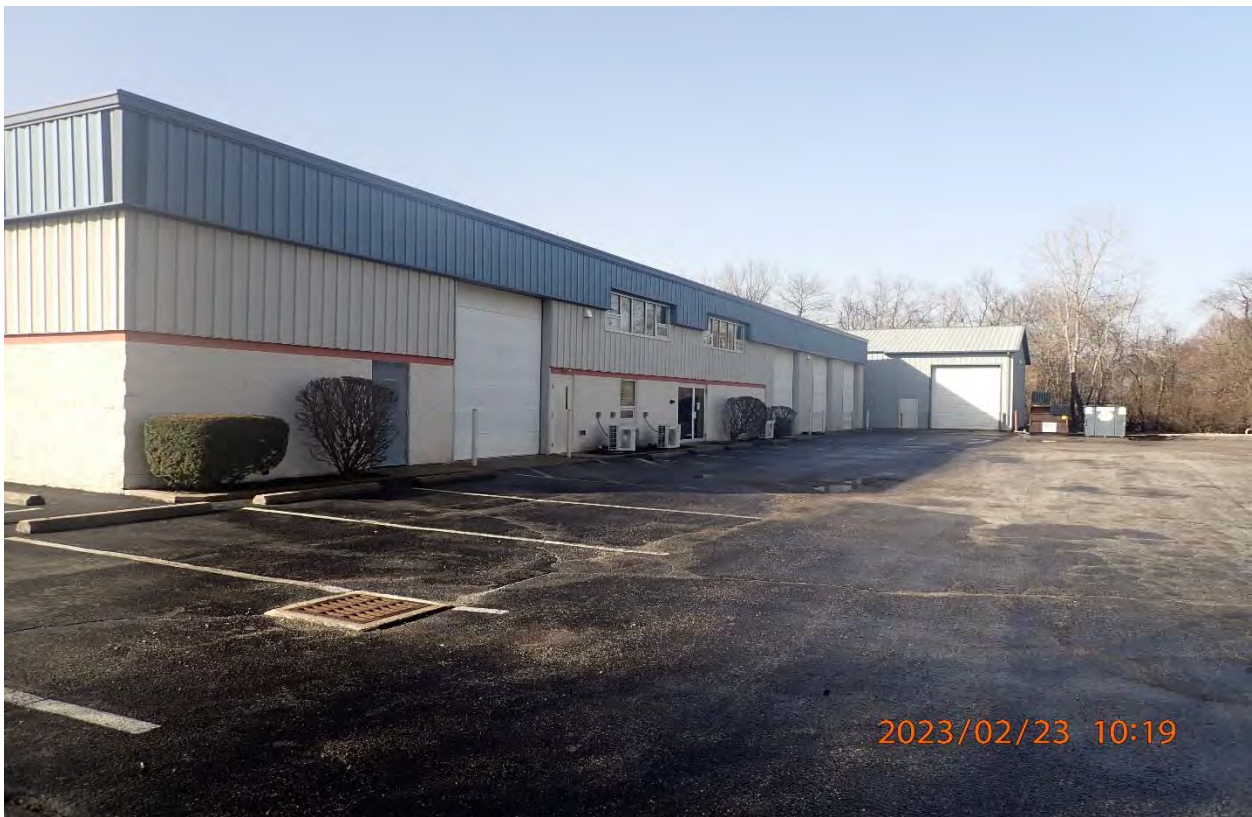
Looking Southwest at the buildings located on the subject property.
