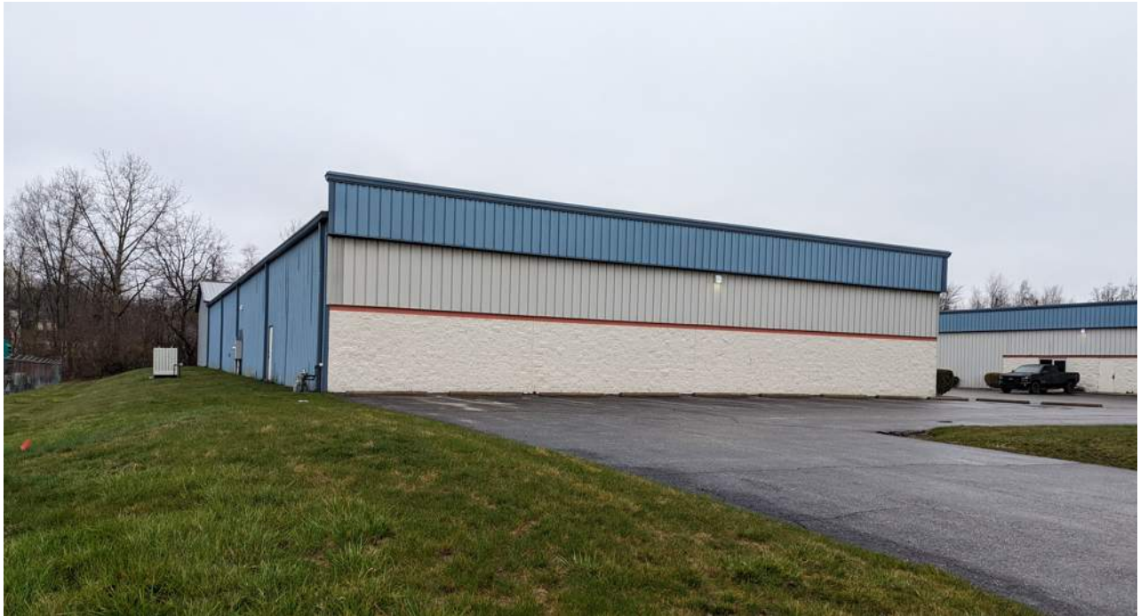
Looking at the south and east elevation of the existing building and the associated parking area in along the east and north side of the building from the southeast corner of the property
