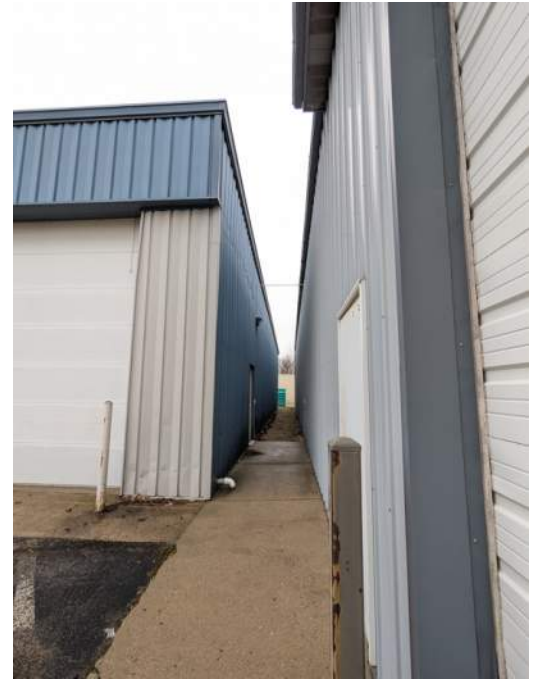
Looking south between the existing buildings on the subject property
