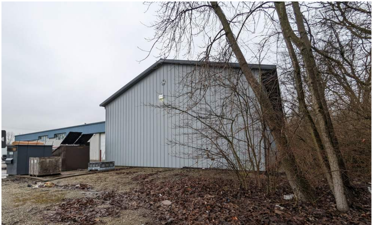
Looking at the north elevation of the existing building at the rear of the subject site and the dumpster area from the southwest corner of the neighboring property to the north
