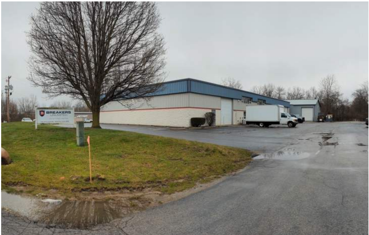
Looking at the north and east elevation of the existing buildings and the associated parking area in front of the building from the driveway of the adjacent property to the north
