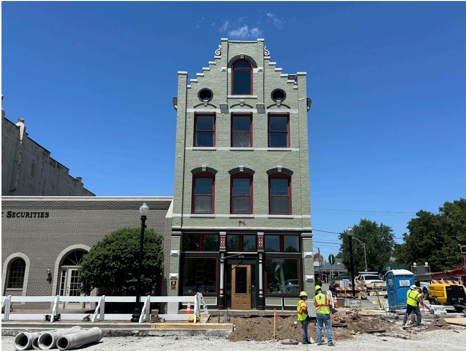
This view of the building faces Conner Street (SR 38).
