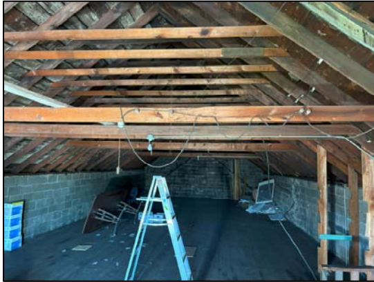
Photo 45: General view of the upstairs storage room
