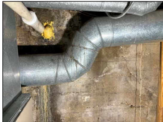
Photo 61: General view of the water stained wall behind the HVAC system
