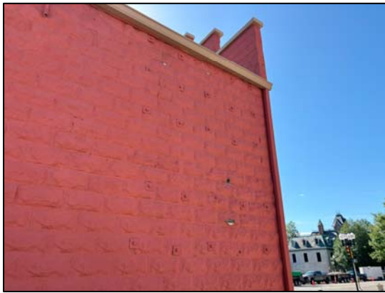
Photo 2: General view of the southwest corner and wall supports
