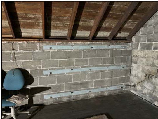
Photo 53: View of wall supports along the southeast wall
