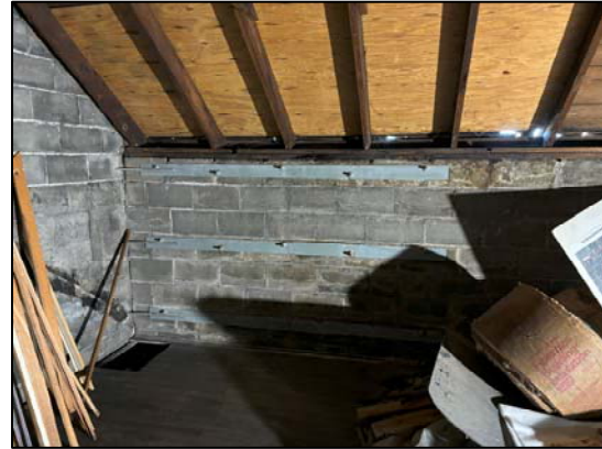
Photo 54: View of wall supports along the southwest wall
