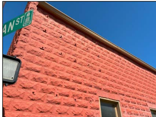
Photo 11: General view of the southeast corner and wall supports
