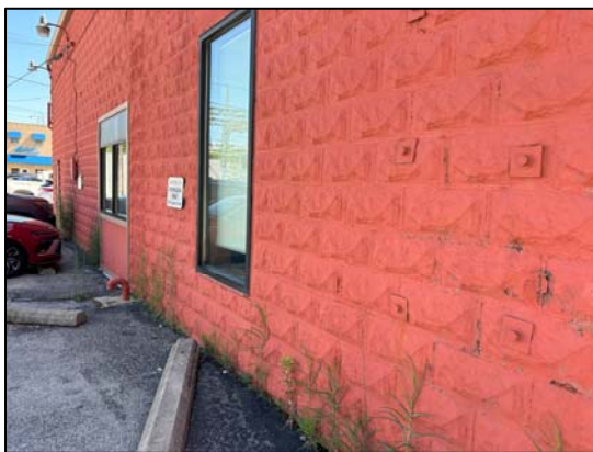
Photo 3: Another view of the southwest corner and wall supports
