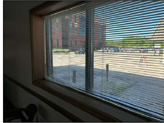
Photo 30: General view of the newer commercial windows
