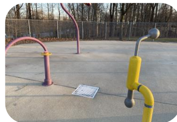
The splashpad's vertical spray elements are 16 years old which is close to the expected lifespan for this type of equipment.
