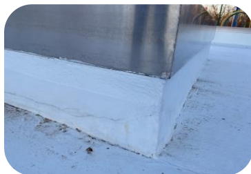
Pool deck cracking that spans over 10 feet in length were observed in multiple places around the pool's perimeter.
