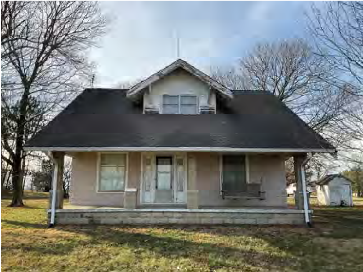
11. Looking W at 1920 farmhouse on Wiseman Farm (IHSSI #057-541-40032, Contributing); Lochmueller recommended rating of Notable/NRHP-eligible
