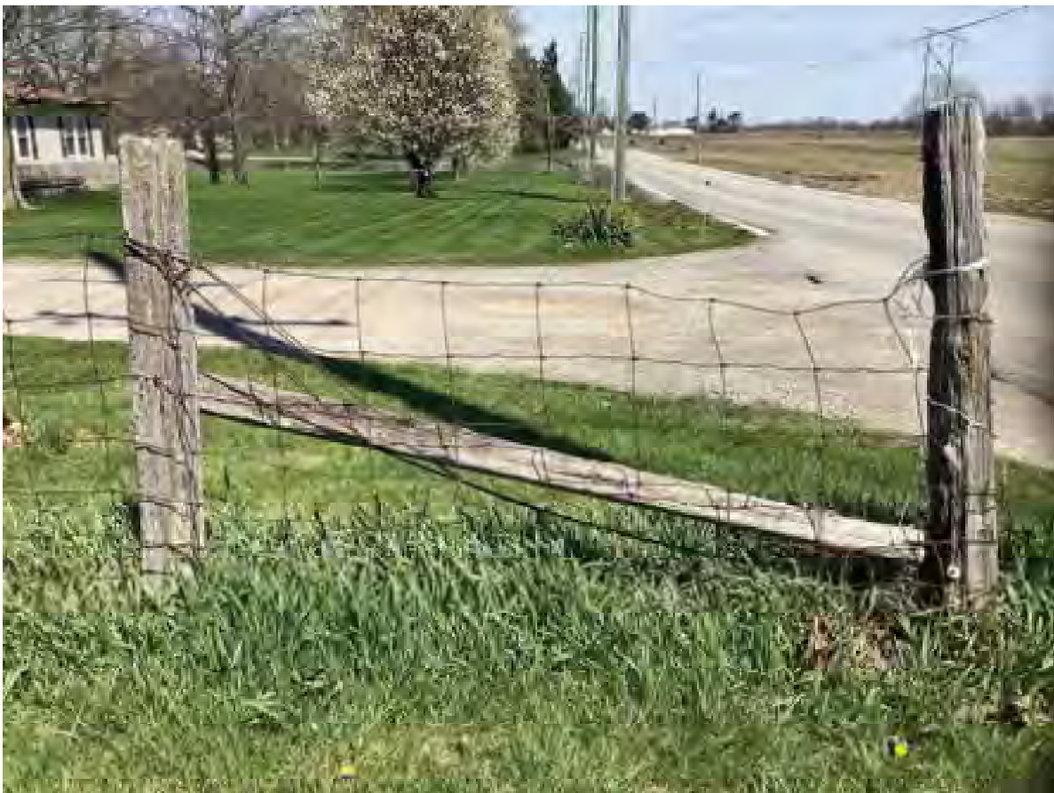
34. Looking N at anchor H frame timber end post on Wiseman Farm (IHSSI #057-541-40032, Contributing); Lochmueller recommended rating of Notable/NRHP-eligible
