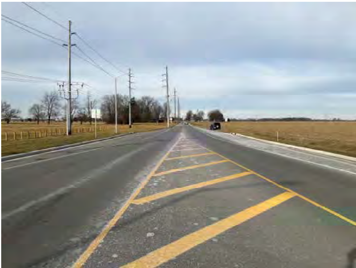
4. Looking N from S end of project limits on Olio Road
