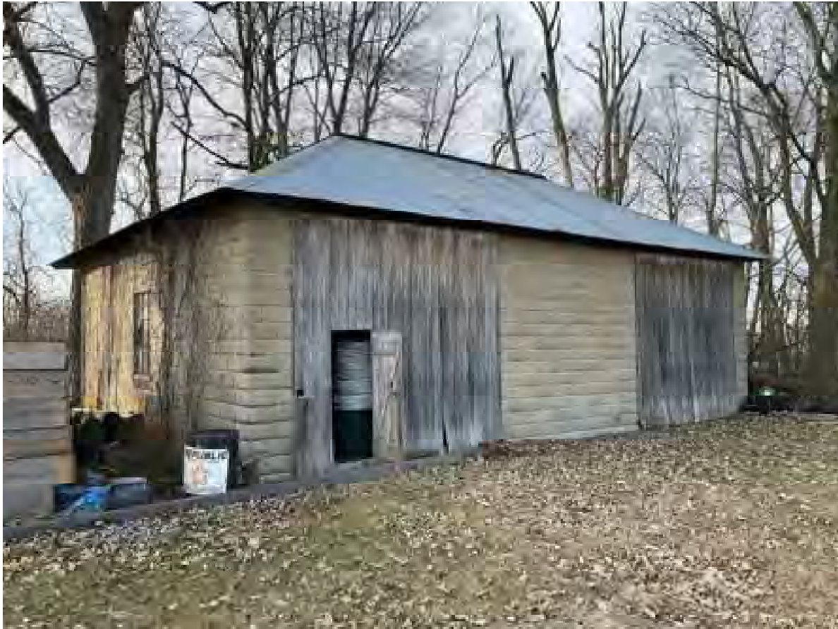
5. Looking NW at c. 1940 garage associated with demolished IHSSI #057-541-40033
