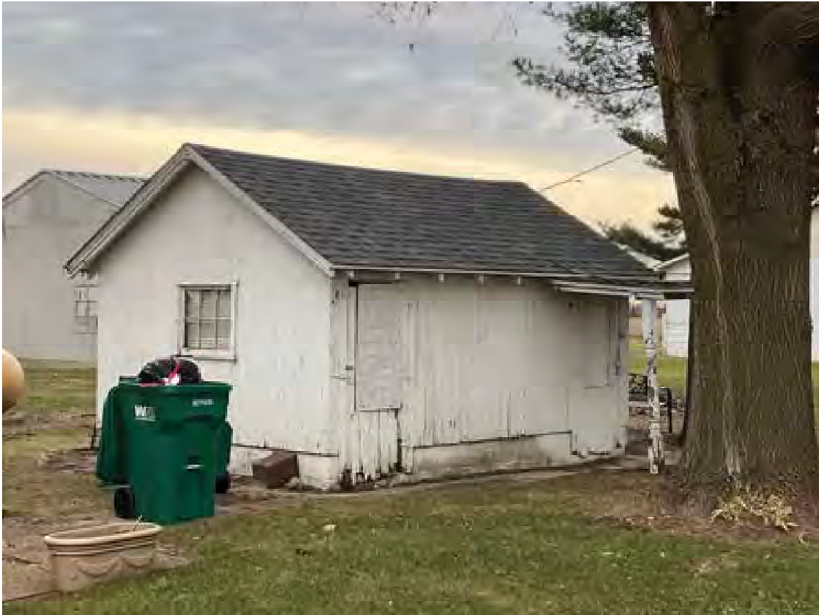
45. Looking NE at shed on Hair-Whitaker Farm (Lochmueller #4, Notable, NRHP-eligible)
