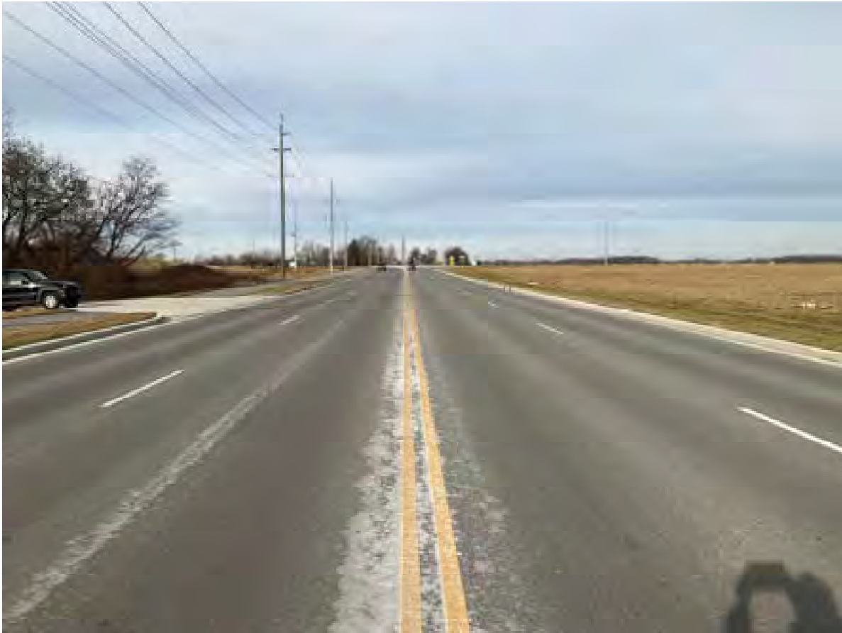
1. Looking N from S end of APE on Olio Road
