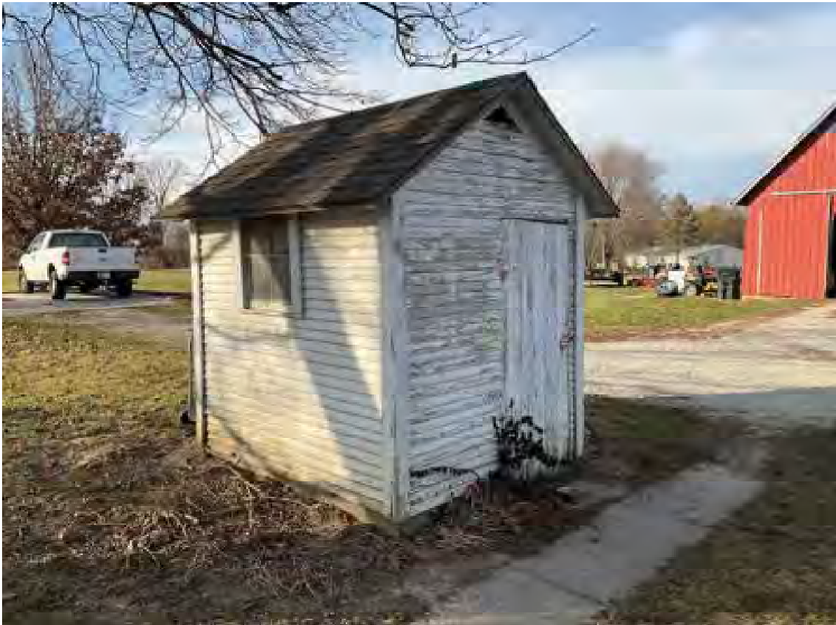
14. Looking NW at well house on Wiseman Farm (IHSSI #057-541-40032, Contributing); Lochmueller recommended rating of Notable/NRHP-eligible
