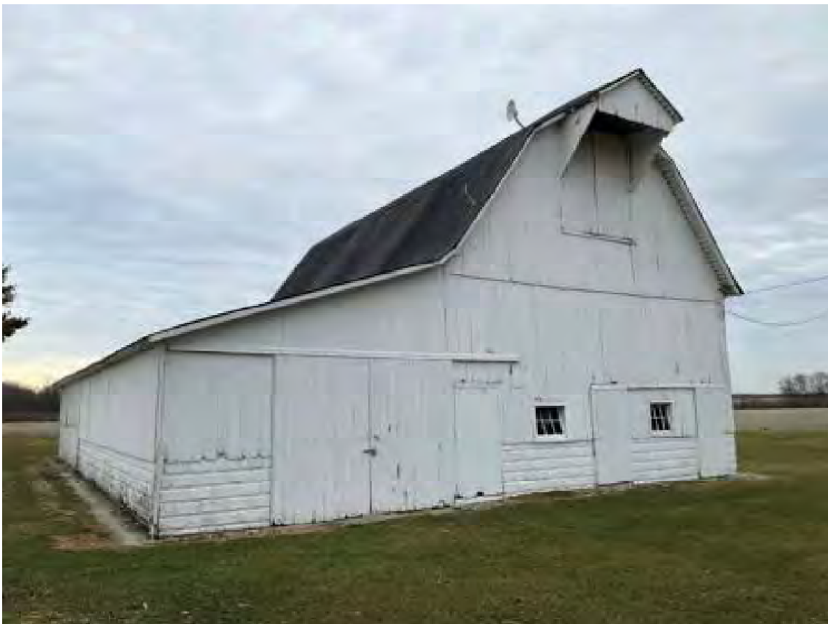
50. Looking SE at gambrel barn on Hair-Whitaker Farm (Lochmueller #4, Notable, NRHP-eligible)
