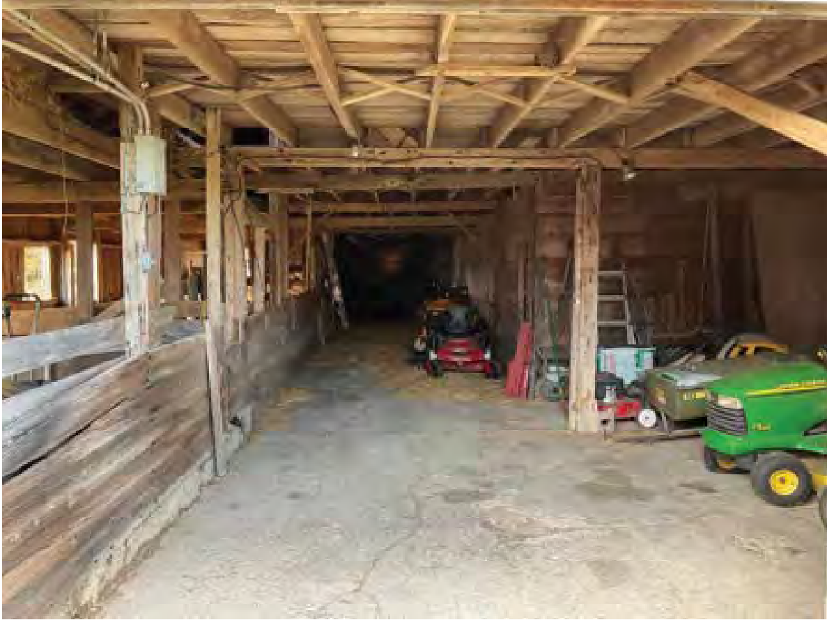
21. Looking N at interior of gambrel barn on Wiseman Farm (IHSSI #057-541-40032, Contributing); Lochmueller recommended rating of Notable/NRHP-eligible
