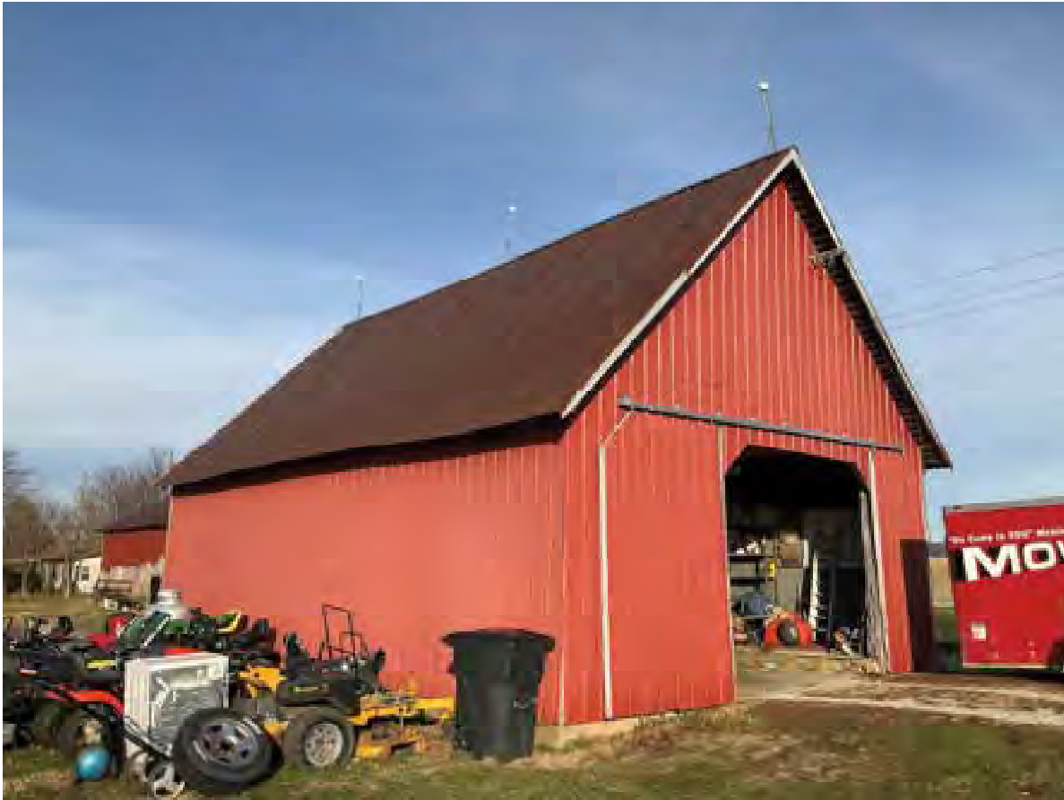
17. Looking NE at gabled barn on Wiseman Farm (IHSSI #057-541-40032, Contributing); Lochmueller recommended rating of Notable/NRHP-eligible
