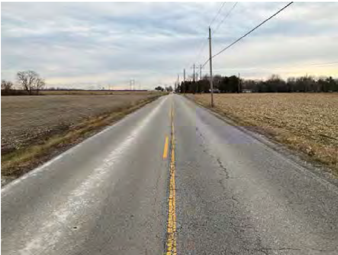
42. Looking S from N end of project limits on Olio Road
