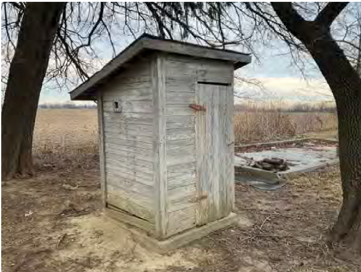
52. Looking NE at outhouse on Hair-Whitaker Farm (Lochmueller #4, Notable, NRHP-eligible)
