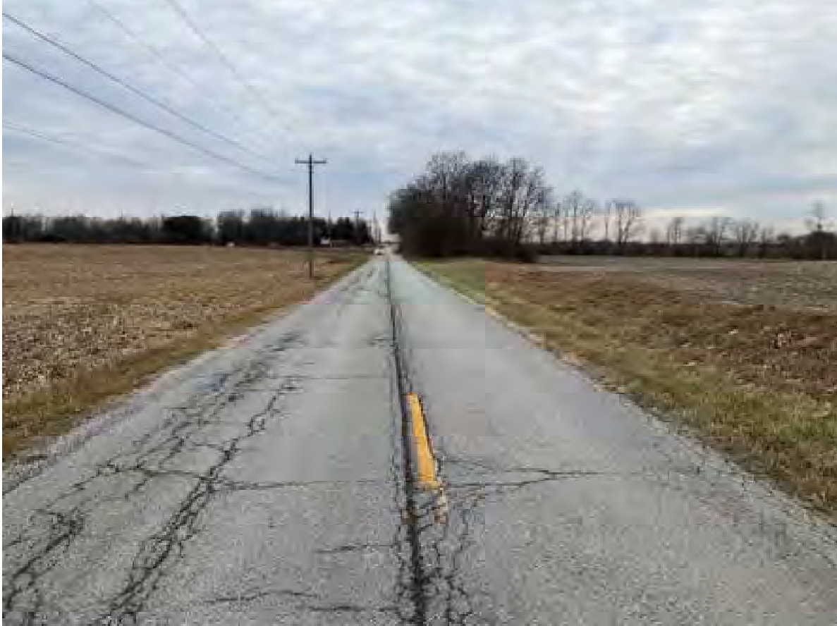
41. Looking W from E end of APE on 156th Street
