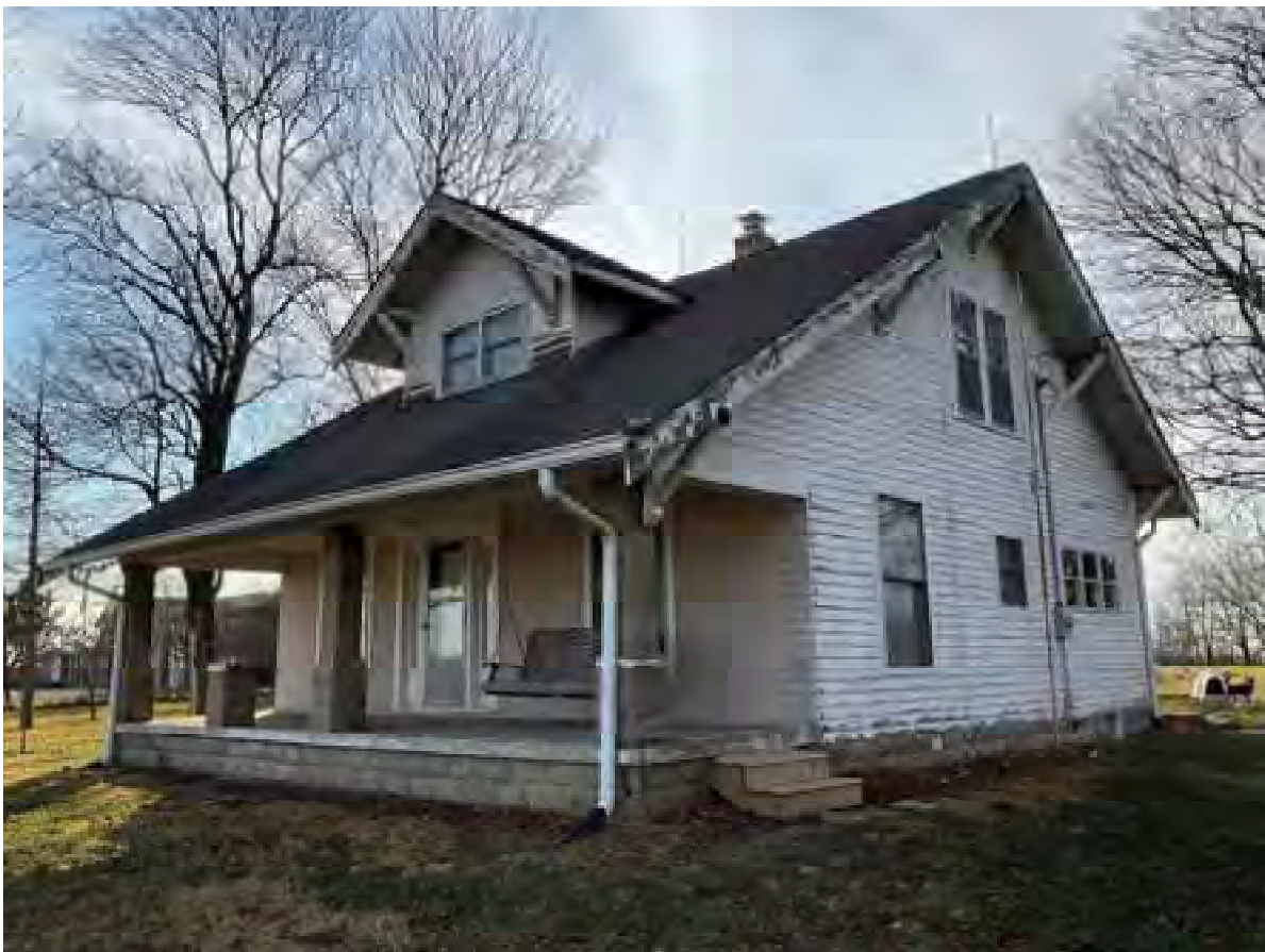
12. Looking SW at 1920 farmhouse on Wiseman Farm (IHSSI #057-541-40032, Contributing); Lochmueller recommended rating of Notable/NRHP-eligible
