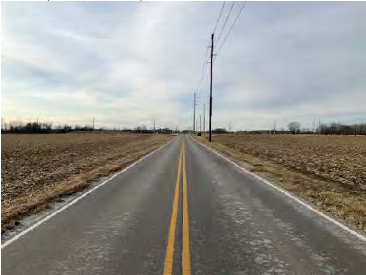
3. Looking W at SE end of APE on 146th Street
