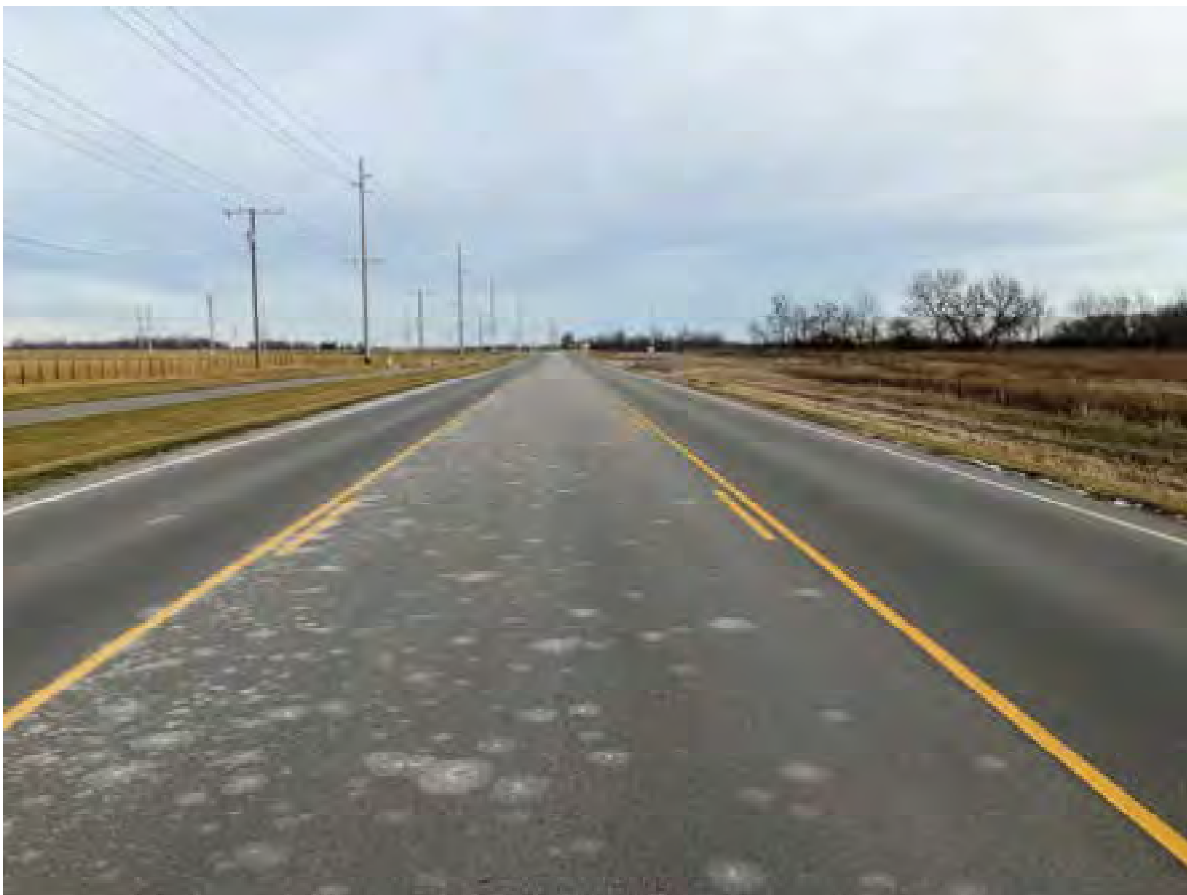
2. Looking E from SW end of APE on 146th Street
