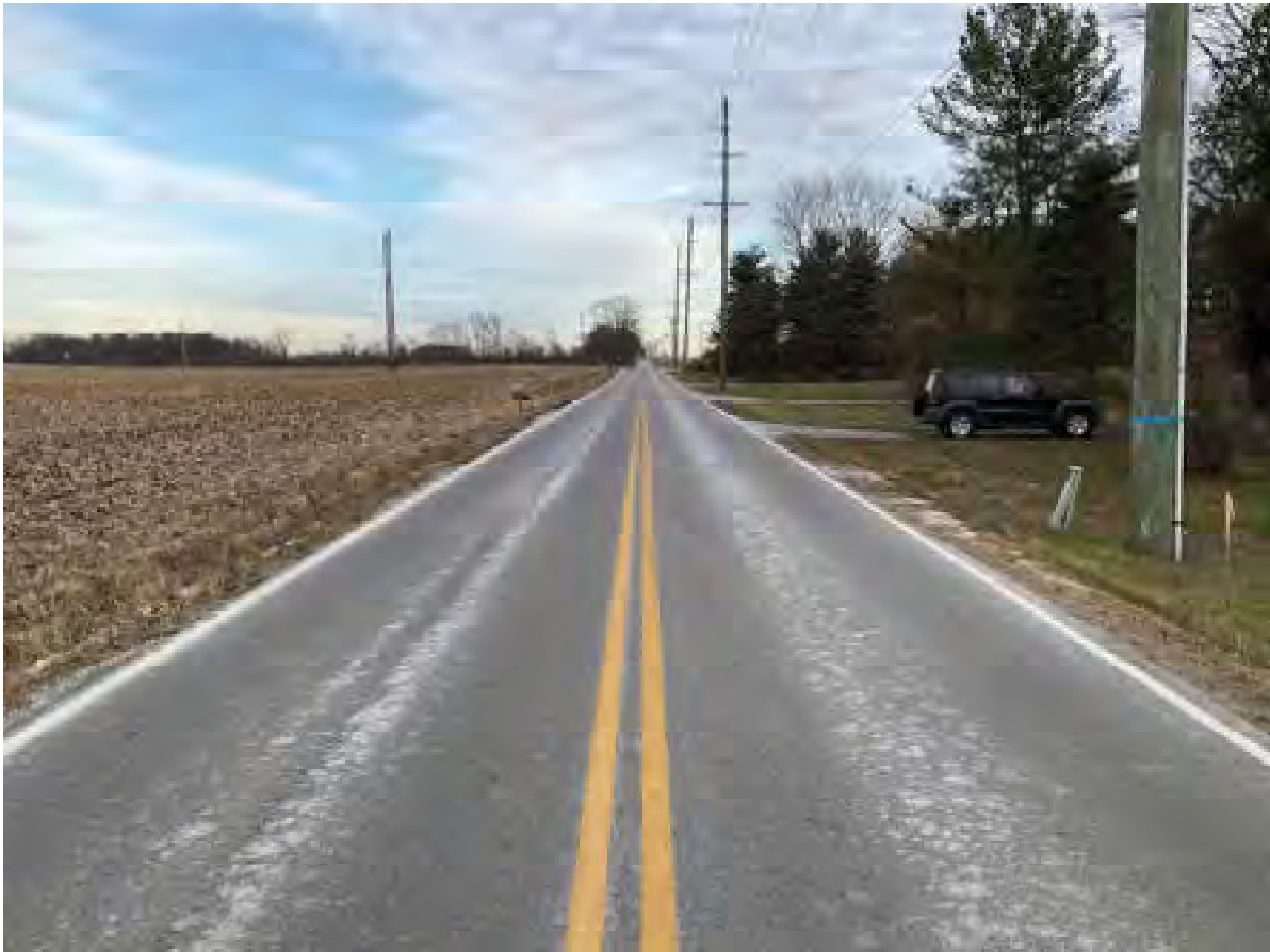
38. Looking E from W end of project limits on 156th Street
