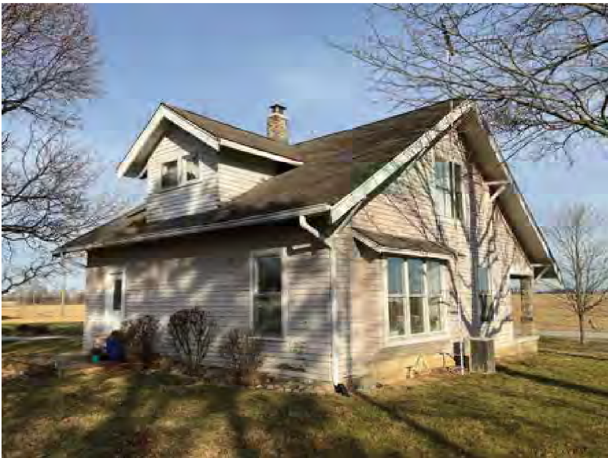
16. Looking NE at 1920 farmhouse on Wiseman Farm (IHSSI #057-541-40032, Contributing); Lochmueller recommended rating of Notable/NRHP-eligible
