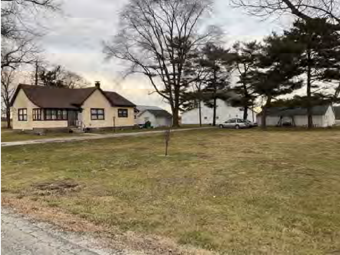
43. Looking NE at Hair-Whitaker Farm (Lochmueller #4, Notable, NRHP-eligible)
