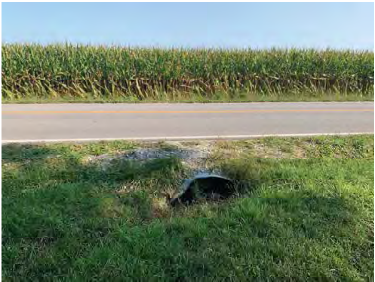
9. Looking north at culvert under 156 th Street- 9/14/22
