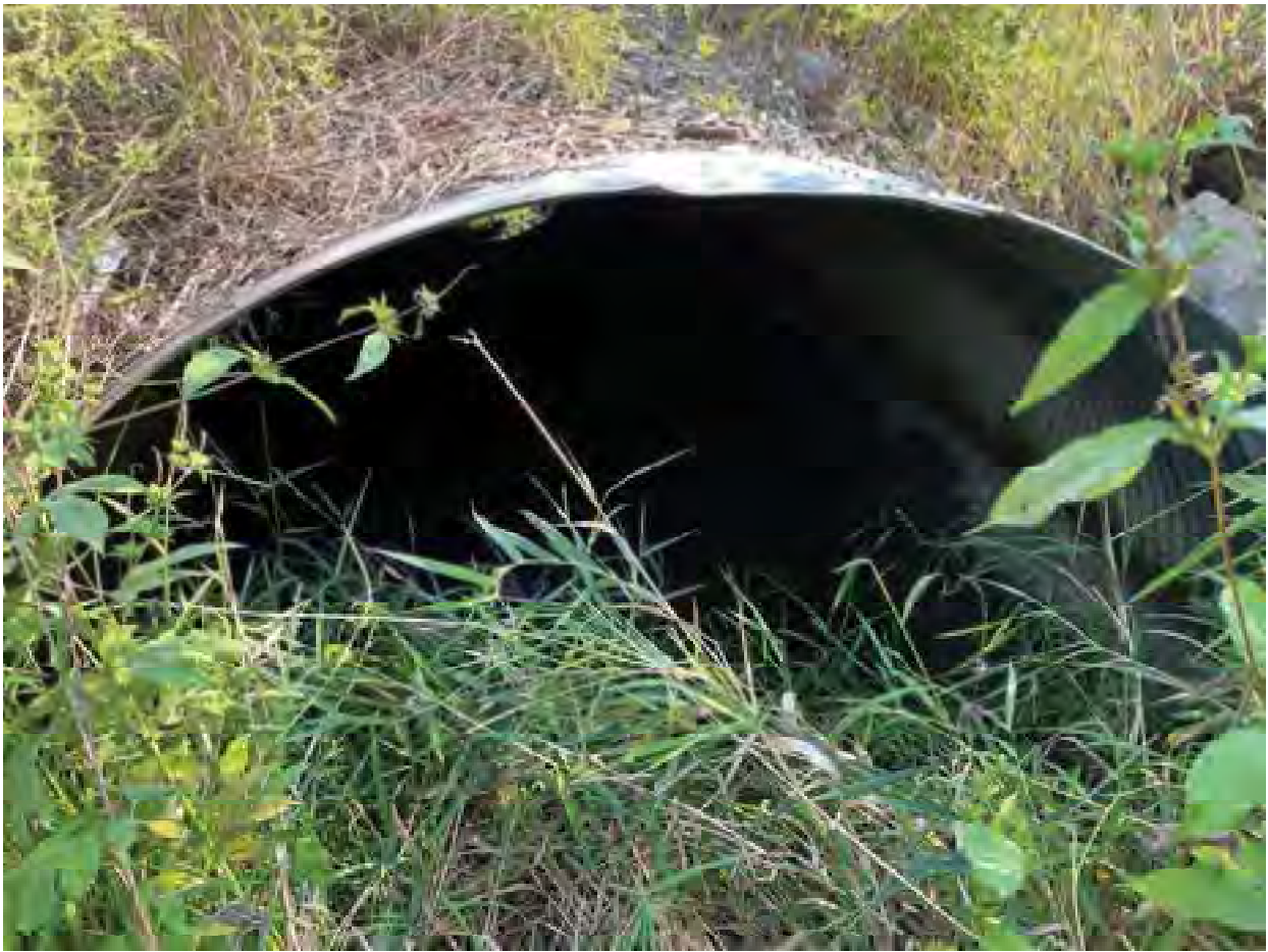
27. Looking northeast through east culvert under 156 th Street- 9/14/22
