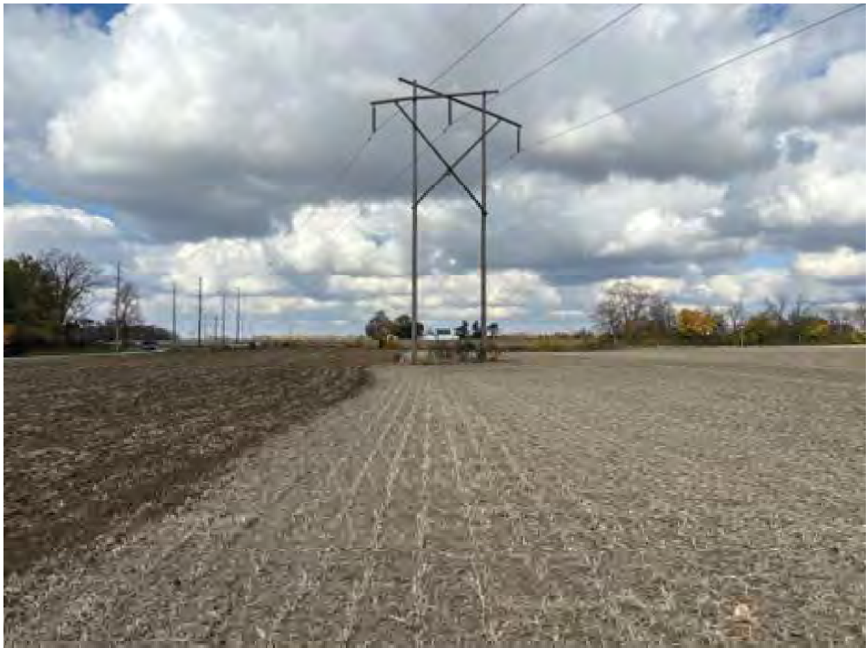
52. Looking north along the east side of Olio Road- 10/30/23
