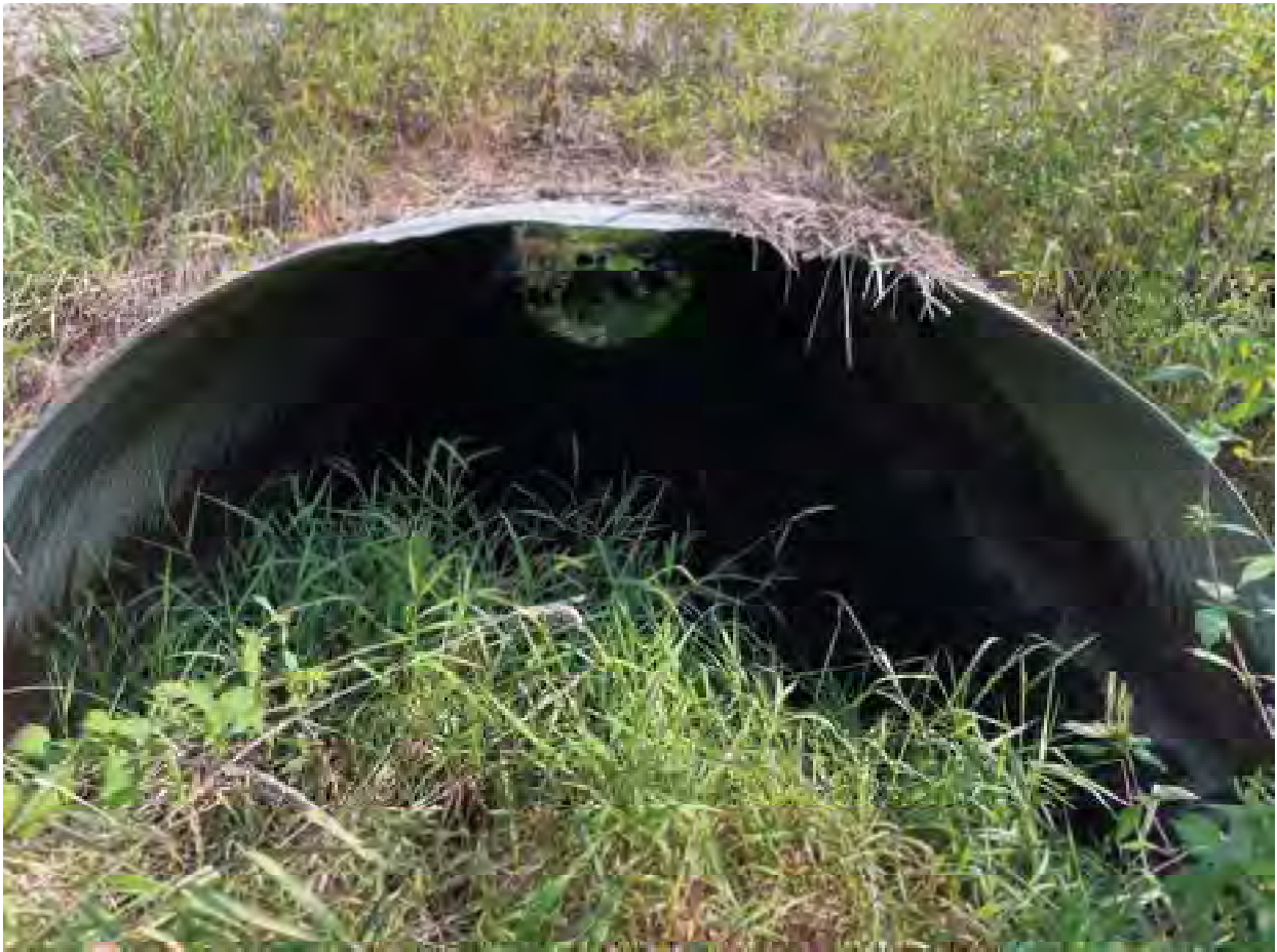
24. Looking northeast through the west culvert under 156 th Street- 9/14/22
