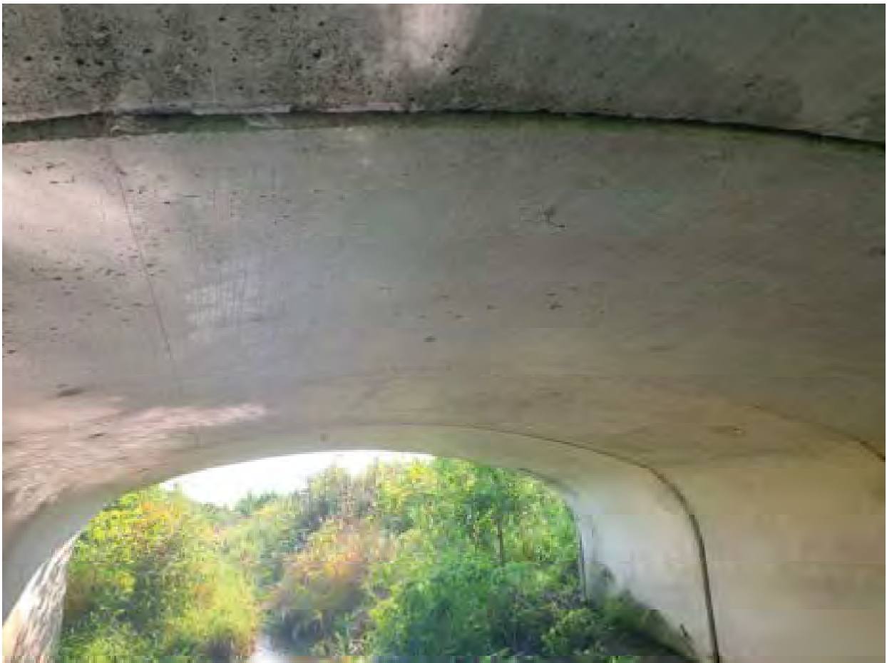
36. Looking east under Bridge #29-00170 over Sand Creek- 9/14/22
