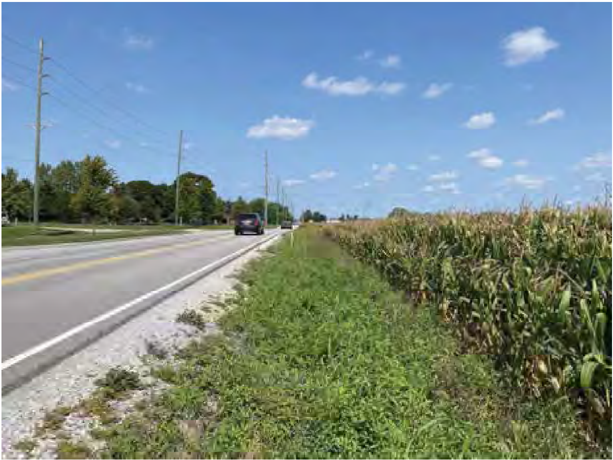
79. Looking north along east side of Olio Road- 9/14/22
