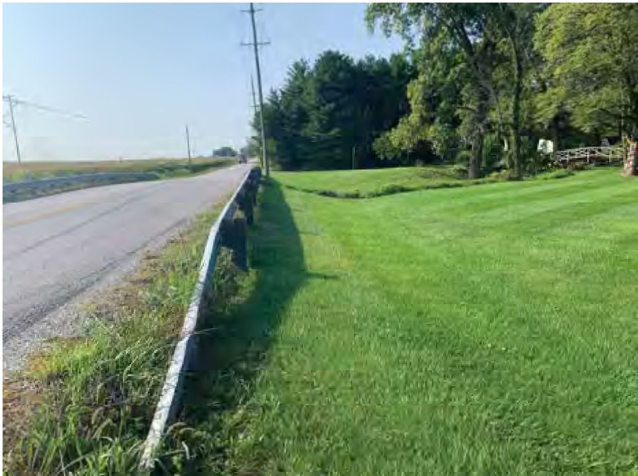
32. Looking south along Olio Road toward Sand Creek- 9/14/22
