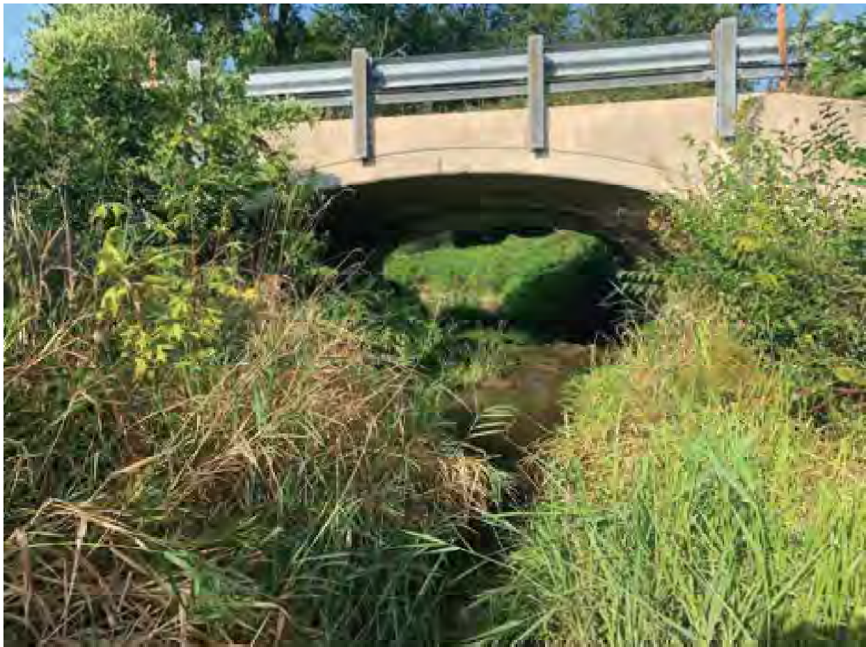
42. Looking west downstream Olio Road at Bridge #29-00170- 9/14/22
