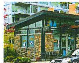
Figure 3: Example of Single-pitch roof
