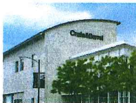
Figure 2: Example of Barrel Roof
