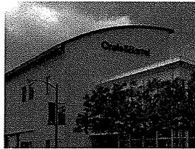
**Figure 2: Example of Barrel Roof**
