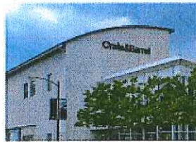
Figure 2: Example of Barrel Roof
