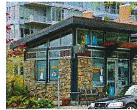
Figure 3: Example of Single-pitch roof
