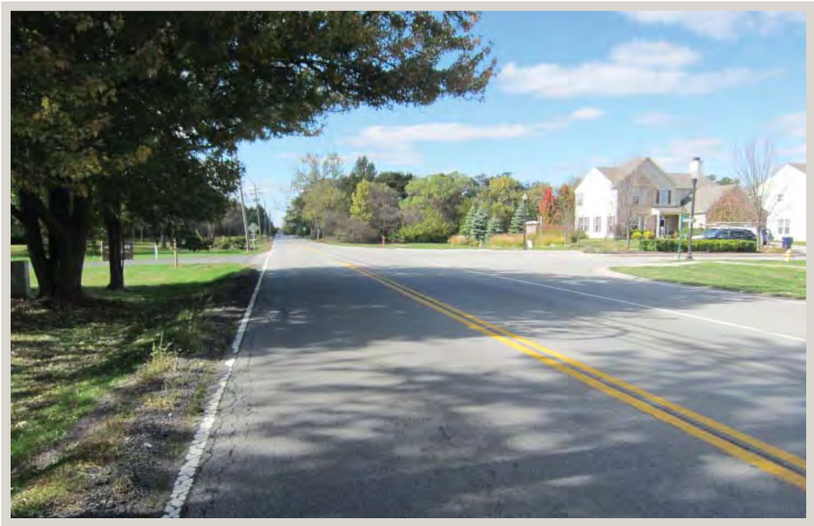
3. Looking northwest along Greenfield Avenue, away from the project area
