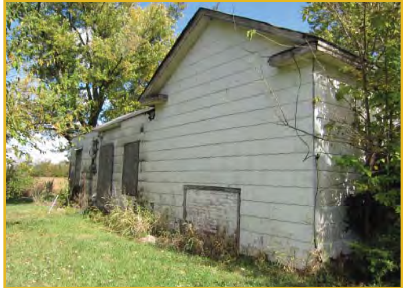
Photo 12: Looking northeast at the west elevation of IHSSI #057-541-30046
