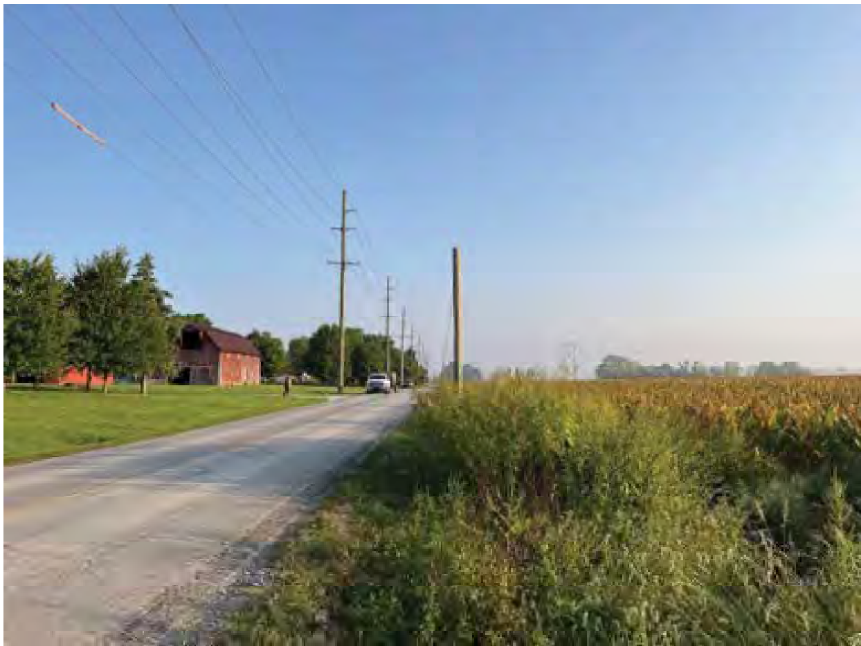
15. Looking north along east side of Olio Road
