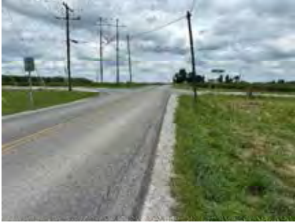
Olio Rd northbound approach, at the intersection.
