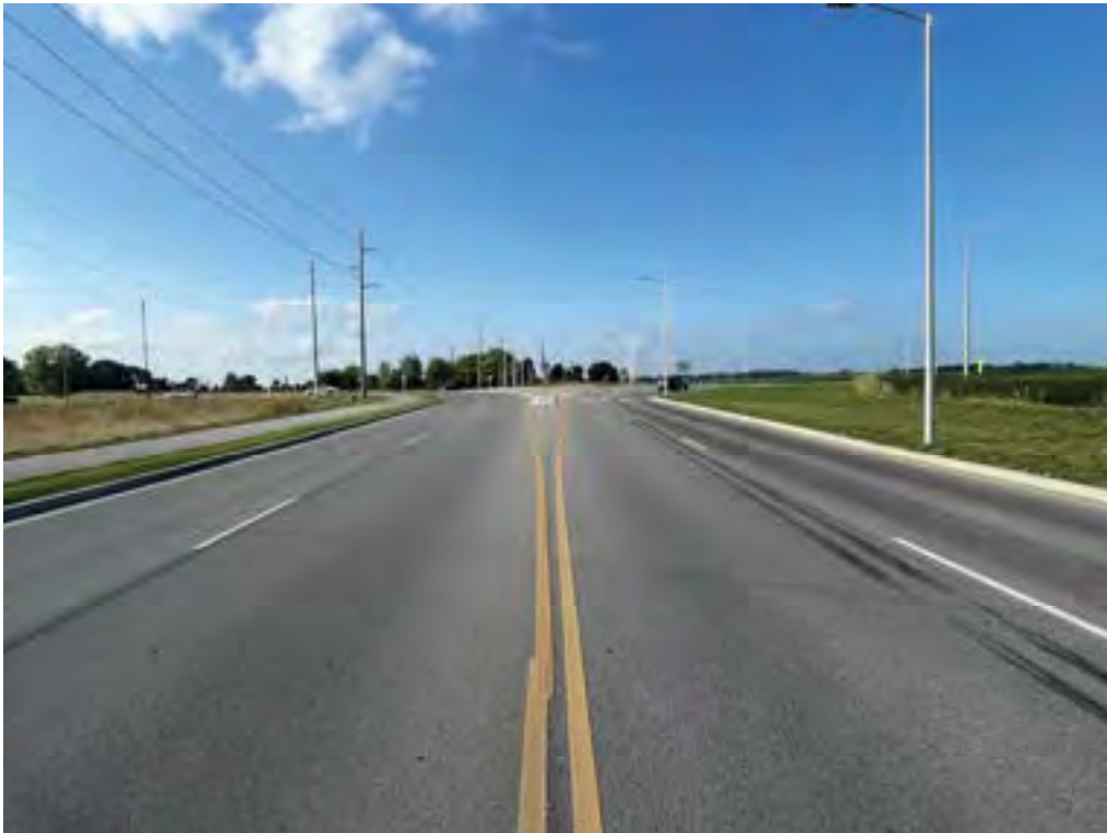
Photo Location 24 - Facing north along Olio Road toward 146th Street roundabout. 8/25/2023
