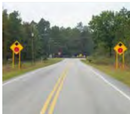
Example of countermeasures on the stop approach. Source: South Carolina DOT
