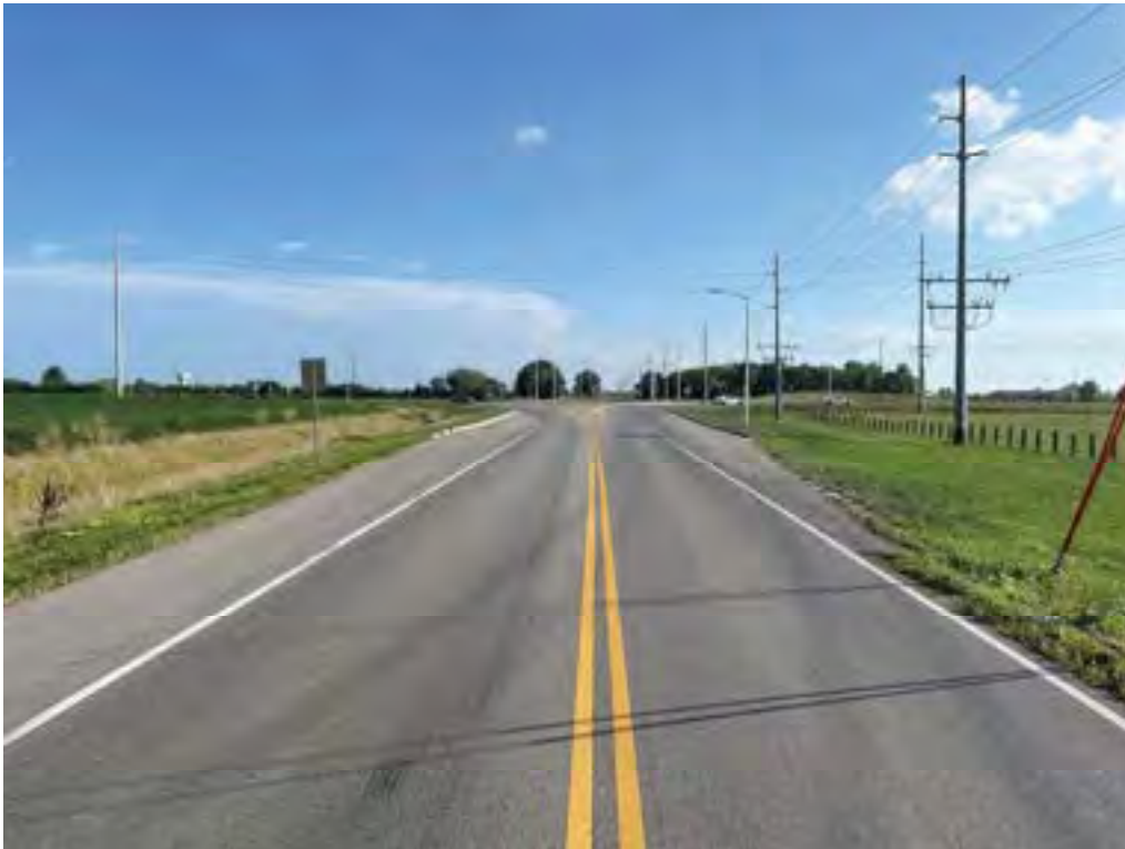
Photo Location 22 - Facing south along Olio Road toward 146th Street roundabout. 8/25/2023
