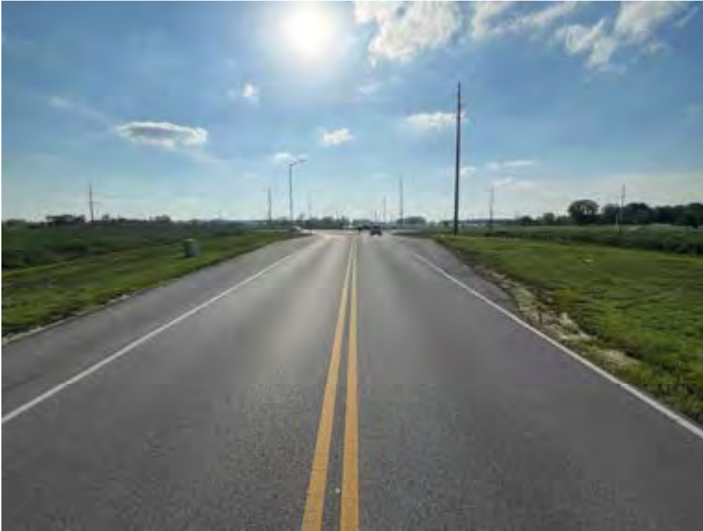
Photo Location 25 - Facing west along 146th Street toward Olio Road roundabout. 8/25/2023
